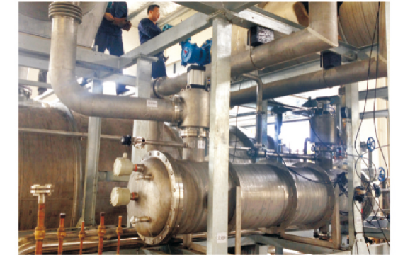
负压或常压热水融冰装置 Negative or ordinary pressure hot water de-icing device
